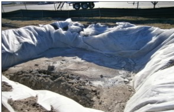
Plate 3-2 Concrete washout area
