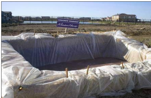
Plate 3-1 Concrete washout area
