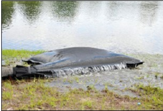
Plate 2-1 Silt Bag with water being pumped through
