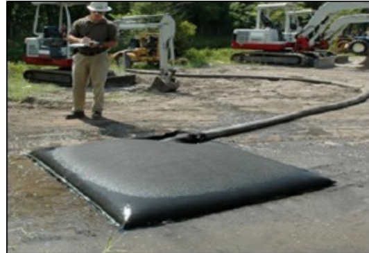
Plate 2-2 Silt Bag under inspection
